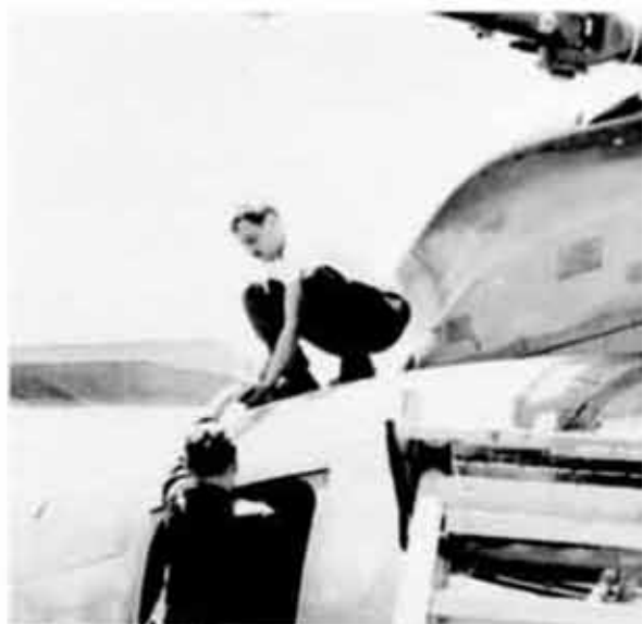
25 Nail the tunnel covers down.
